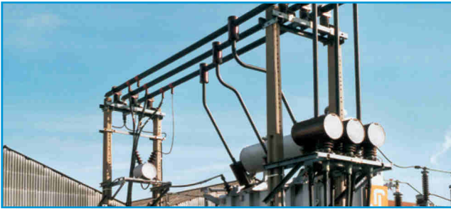
GASLINK® SF 6 insulated busbar system
